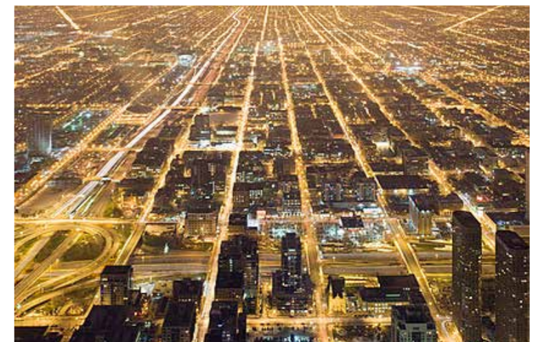
Smart grid: Chicago's regular street plan was laid down by the city's founders, with eight streets to every mile running westwards from Lake Michigan and 16 aligned north-south.
